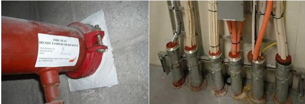
Figure 4: Fire Stopping Through Walls and Floors
